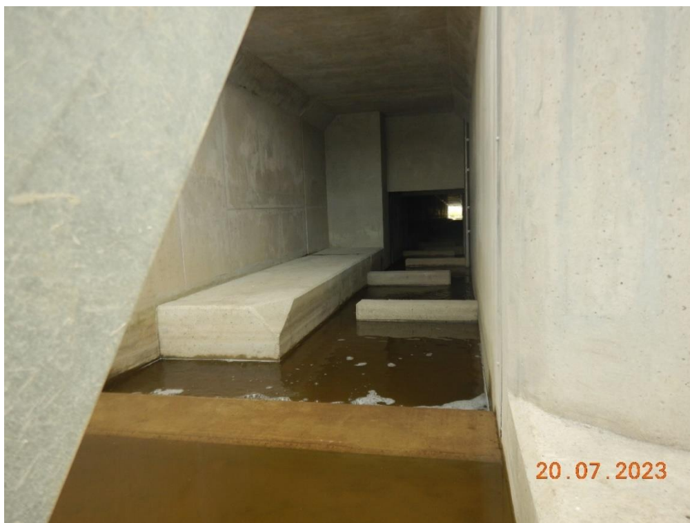
Phot.6. Thresholds constructed in the adit (item no. 53 of EMP).
