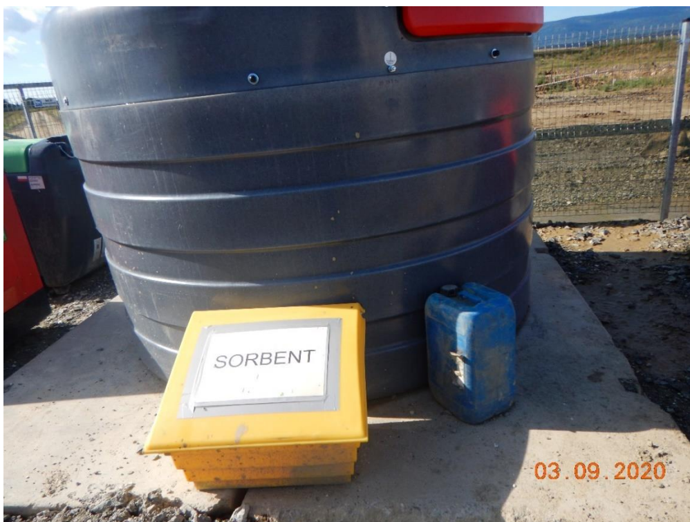
Phot.4. Vehicle refuelling point equipped with sorbent (item no. 80 of EMP).
