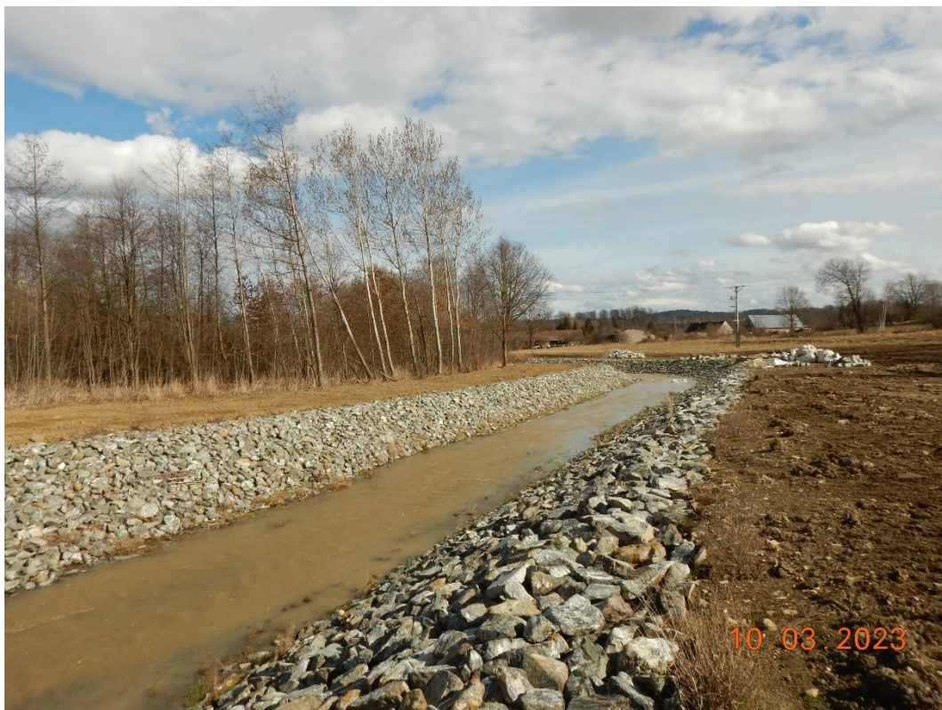
Phot.10. Rip-rap made on the slopes of the new Duna channel (item no. 45 of EMP).
