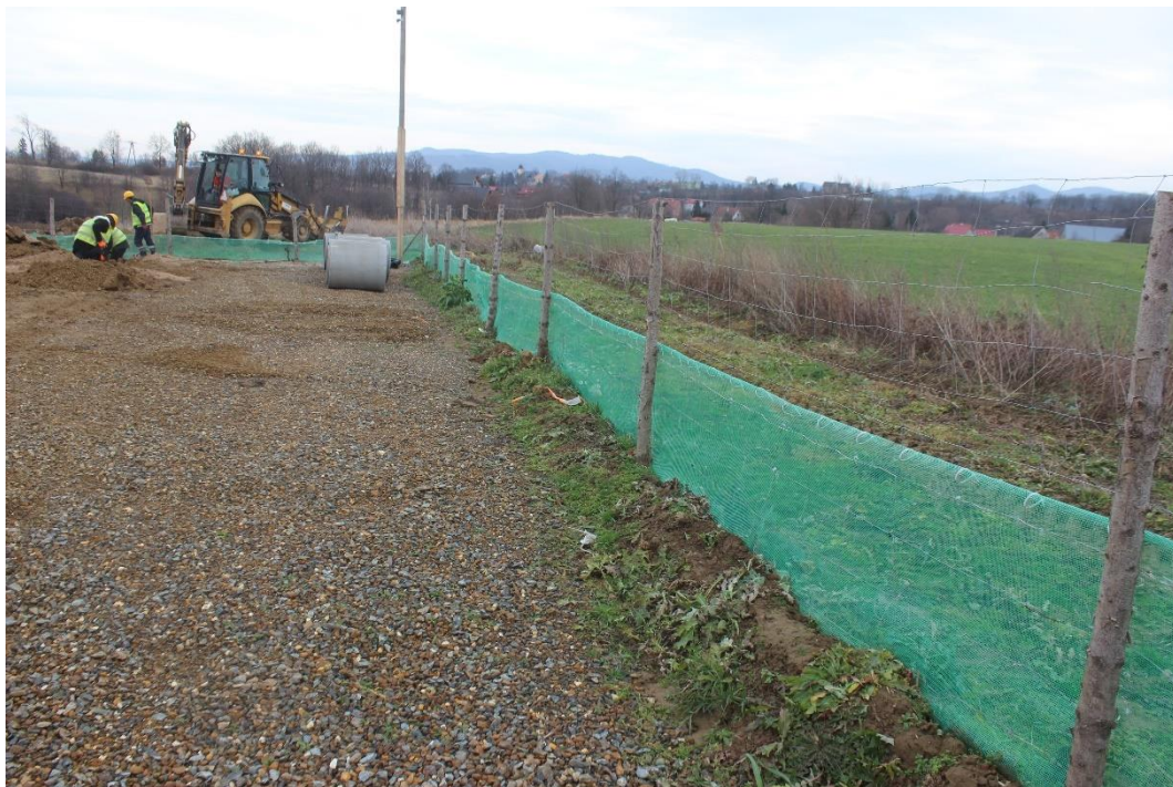
Phot.9. Protection of construction site facilities against access of small animals (item no. 31 of EMP).
