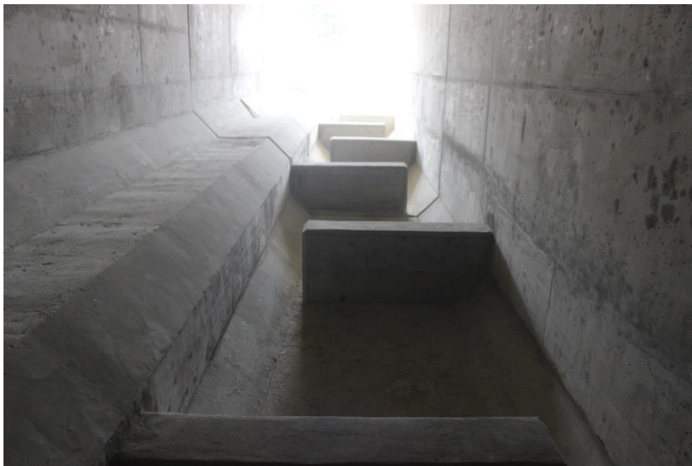
Phot.5. Thresholds constructed in the adit (item no. 53 of EMP).
